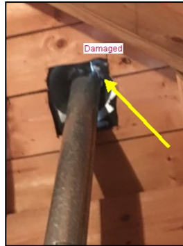
Water heater vent boot
